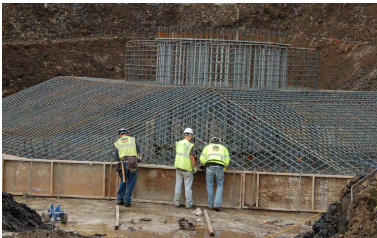
Inset. 5.3-34 Turbine foundation construction
