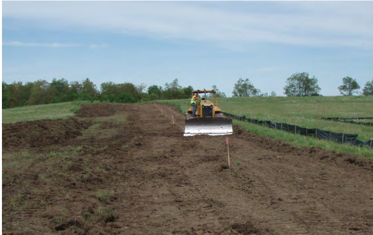
Inset 5.3-33. Construction of Access Roads (topsoil stripping)
