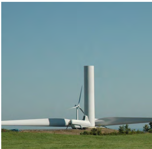
Inset 5.3-35. Turbine laydown and assembly
